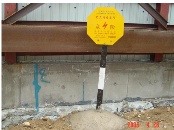
F: Warning sign of "High Voltage Cable Beneath" is erected in the site.
