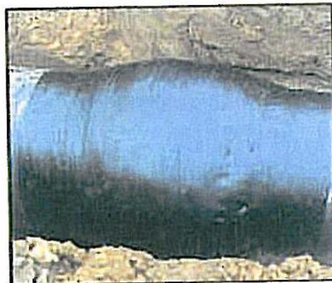
Picture 2: completed wrapping
