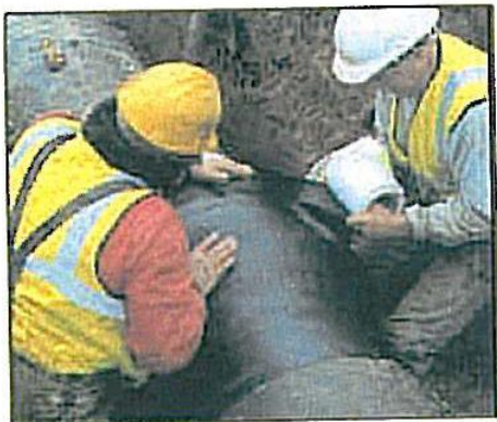
Picture 1: Wrapping in process
