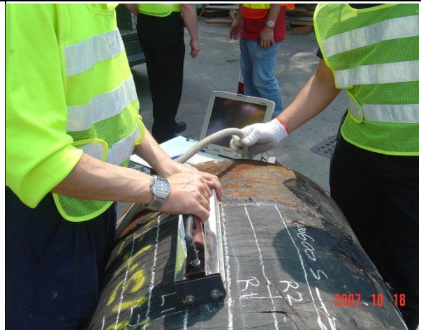
B: Ultrasonic thickness measurement at bare joint area
