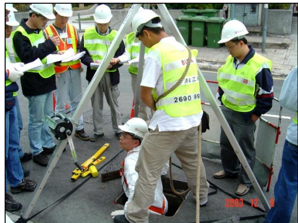
Figure 3.6 Safety Training on Site
