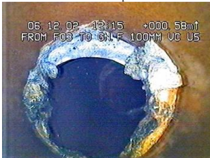
C: Encrustation- Heavy encrustation
