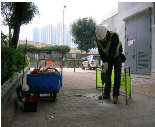
E: Hole drill for gas leakage detection.
