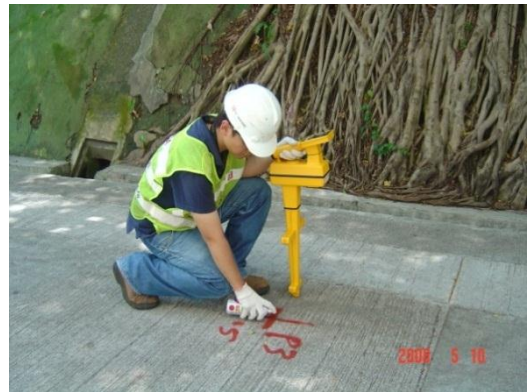
B: Finding out the alignment of the mains before leakage detection.
