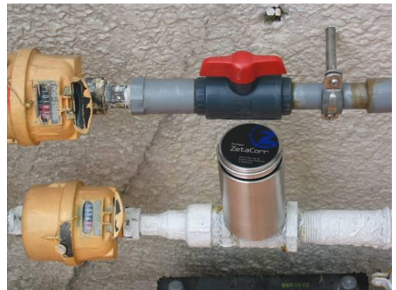
F: A noise logger is installed to collect leak sounds.
