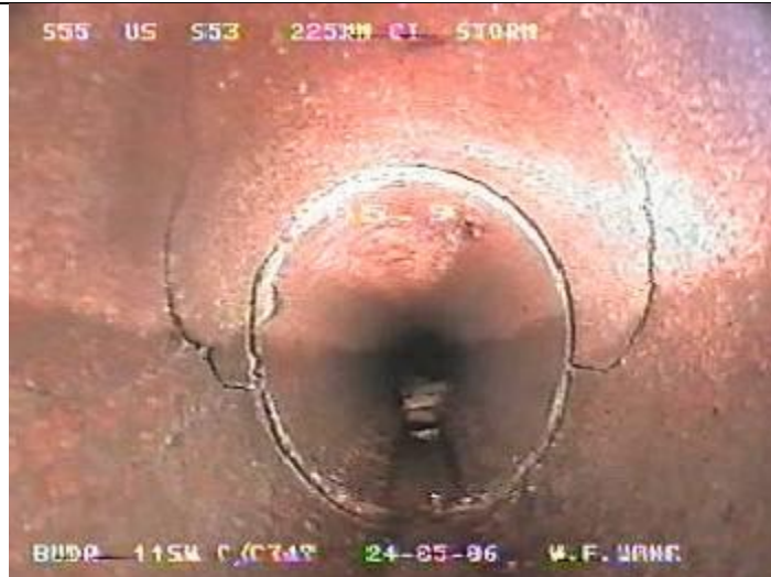
D: Circumferential Fracture from 9 to 3 O'clock
