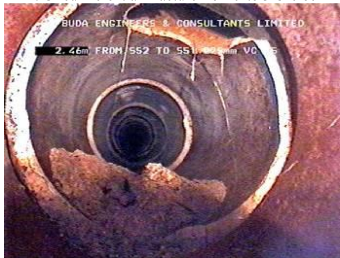
E: Hole at 12 to 01 O'clock
