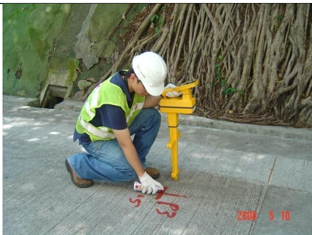
E: Marking the location of the utility detected.
