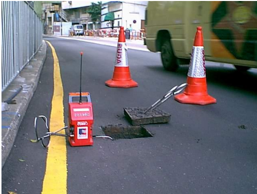
C: The LNC set is collecting the sounds of the pipe.
