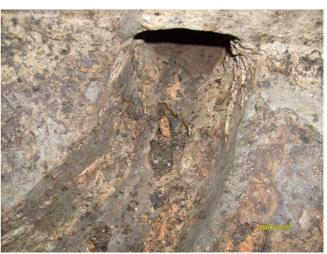
Fig. 4 Other condition: Invert was found broken. 圖四. 其他狀況: 行水破裂
