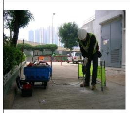
E: Hole drill for gas leakage detection.
