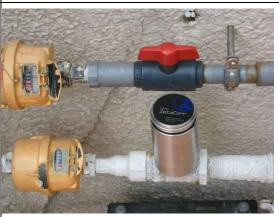
F: A noise logger is installed to collect leak sounds.
