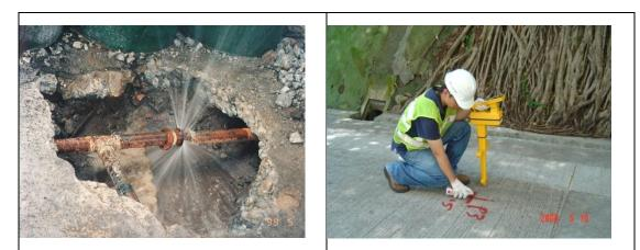
A: Water burst from a deteriorated water B: Finding out the alignment of the mains main. before leakage detection.
