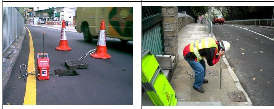
C: The LNC set is collecting the sounds of D: Manual listening by experienced the pipe. operator gives a reliable result.
